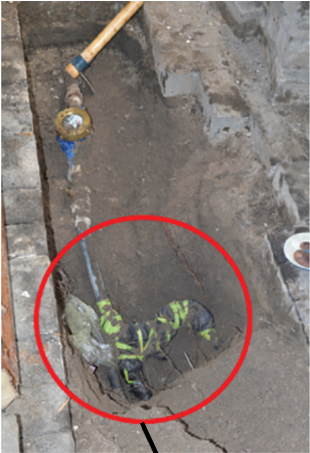
Underground bypass before meter
